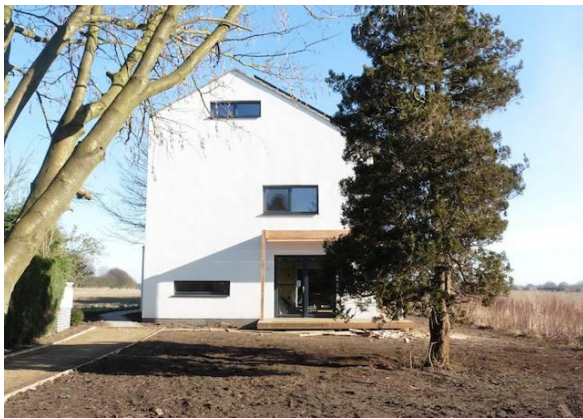
Approach to the building from the west side.
