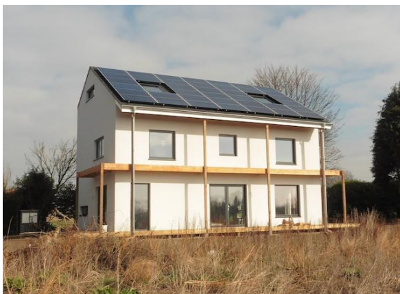
South-west view showing the solar array.
