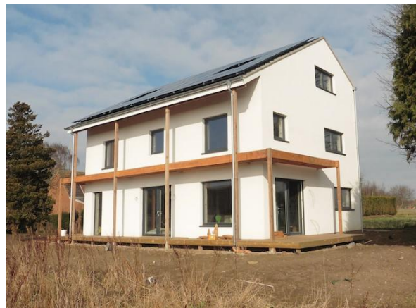
South-east view of the house showing the shading to the south side and asymmetric roof.
