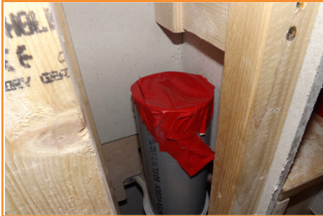
3.2.1 End of waste temporarily sealed after DIRGO removed
